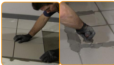
Install the floor finishing (ceramic or wood)
