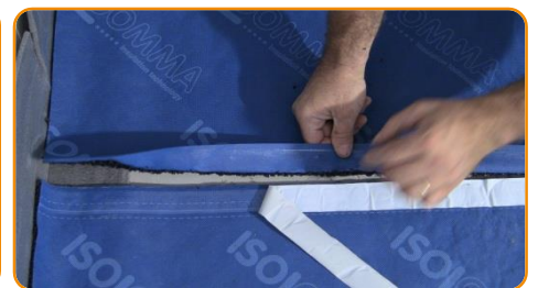
Joint two adjacent mats using the pre-built adhesive tape and following the dashed lines
