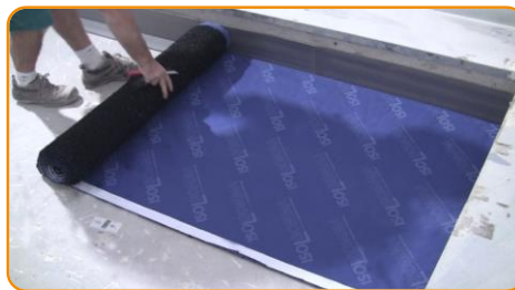
Install the acoustic mat with rubber granules facing down
