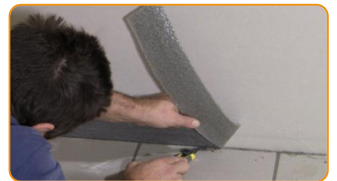
Cut the exceeding part of the edging strip
