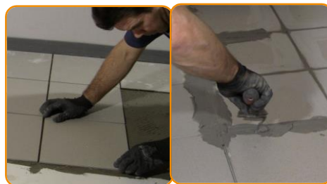
Install the floor finishing (ceramic or wood)
