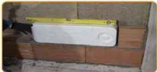
Lay the Sylencer horizontally on the mortar layer.
