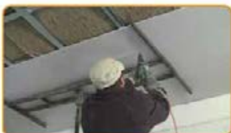
Fix the gypsum board by screwing
