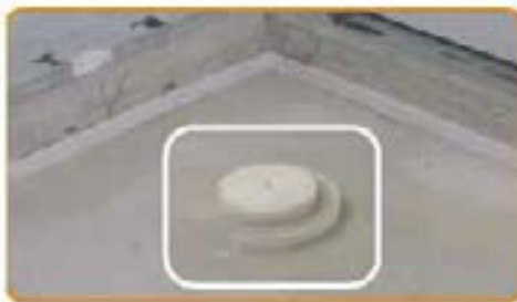
Fix the Profyle Flat 5 around the bottom of the surrounding walls
