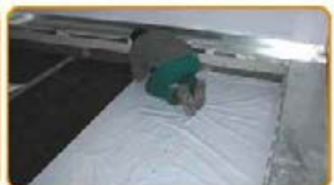
Apply polyethylene layer with as protection film.
