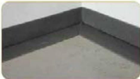
Insulate the acute corners with the "Profile" strip by cutting it as shown in the drawing.
