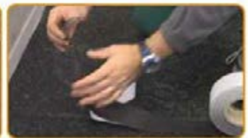
Tape all the Sylcer jointing borders with the Stik tape
