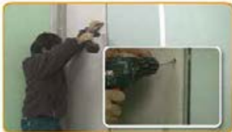
Cover the insulation layer by screwing the second gypsum boards on the metal studs
