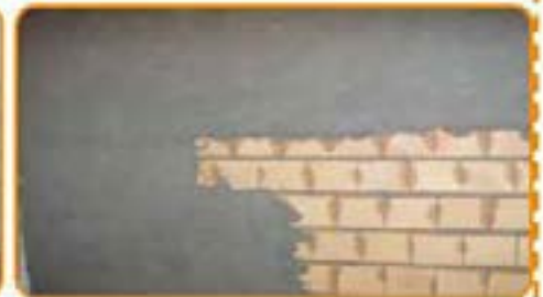
Realize the final plastering.
