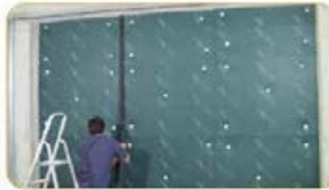
Remove the protective film and seal the joints of the rolls, wall panels and Profyle
