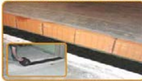
Lay the under wall strip in the dry floor and build the wall.
