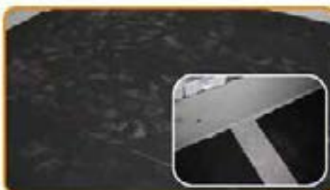
Lay down the insulation layer. Seal the roll border by using the adhesive stick tape.
