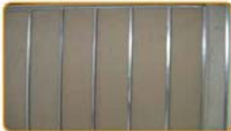
Fix the gypsum boards on one side
