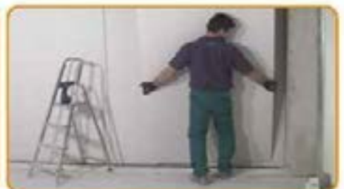
OPZION - DOUBLE GYPSUM BOARD - To improve structurally the dry wall apply a second board
