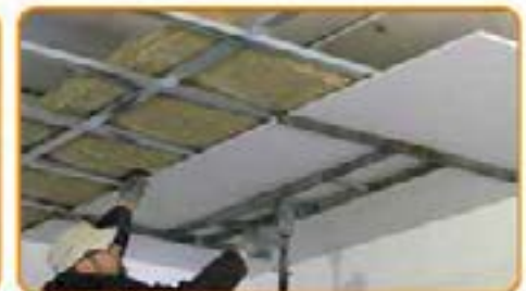
Lean the gypsum board to the metal frame
