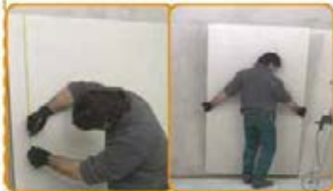
On each Rewall panel mark the holes points placed as per the drawing here shown
