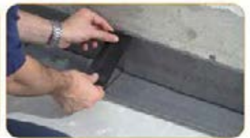
Remove the protective film and seal the joints of the rolls, wall panels and Profyle
