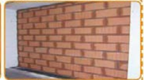
Build up the wall by caring to joint the blocks with mortar on both vertical and horizontal joints.
