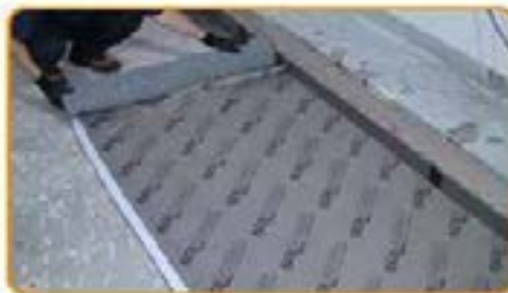
Lay down the insulation layer on the floor surface with the rubber granules turned on the bottom floor side.
