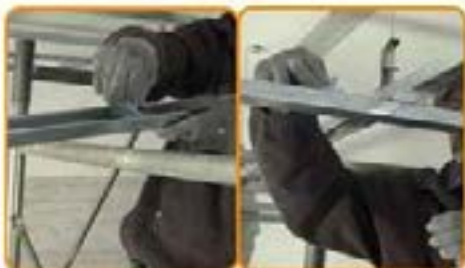
Fix the metal stud of secondary grid to the primary grid with the appropriate connector
