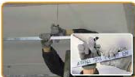
Fix to hangers the metal studs of primary grid
