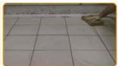
When the grouting starts to solidify the ceramic clean can be done.
