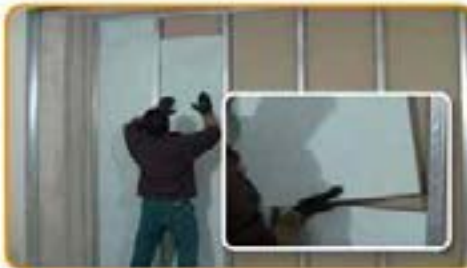
Insert the Trywall panel
