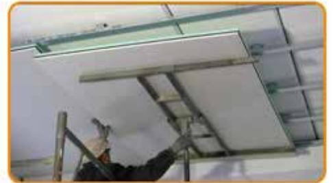
Lean the Rewall panel to the metal frame
