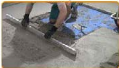
Melt the screed
