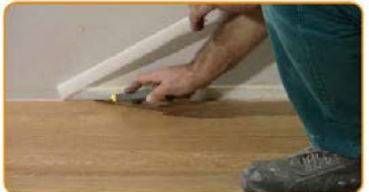
When the flooring application is completed, cut the exceeding part of the edging strips.
