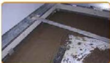
Melt the screed
