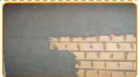
Realize the final plastering
