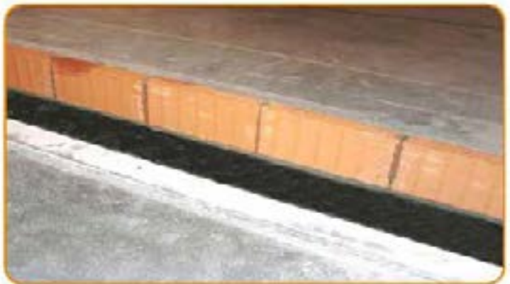
Over the Stywall lay down a plaster bed in order to start to built up the wall
