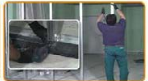
Fix the vertical metal studs on the ceiling and bottom guides by screwing
