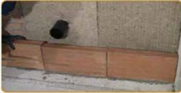
Start to built the wall
