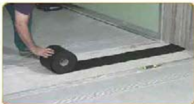
lay the under-wall strip.
