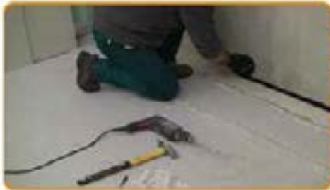
Lay the under wall strip
