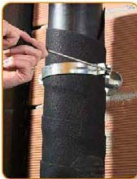
Insert the pipe in the proper casing.
