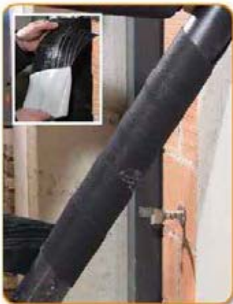
Remove adhesive film and glue the product around the pipes.
