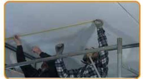
Calculate the distance of the metal studs of 50 cm and fix the acoustic bracket every 80 cm
