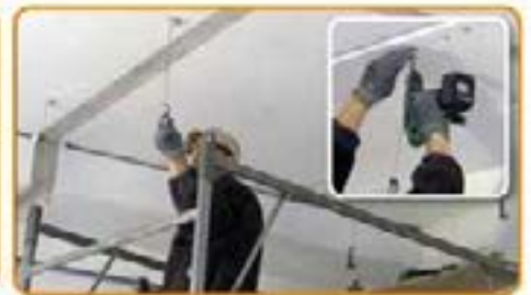
Mark and fix the acoustic hangers
