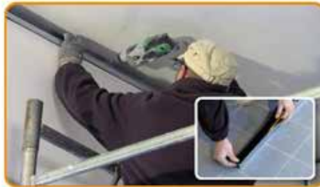
Glue the adhesive strip Stywall S3A to the metal studs and fix them along the upper perimeter of the room
