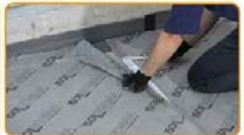
Seal the roll jointing borders by the adhesive flap available on the roll border. To do it properly follow the dotted end continues lines indication.
