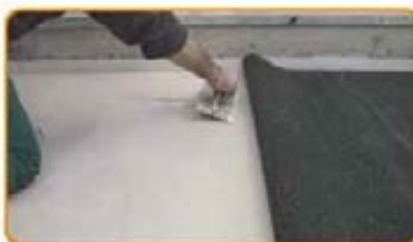
Spread a thin layer of adhesive onto the floor, then glue the Sylcer
