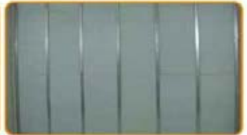
Complete the insulation application
