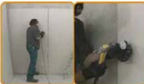
Proceed drilling the holes by a 10 mm driller and apply the nails
