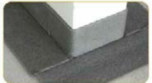
Apply the Profyle all along the walls room perimeter, as shown in the drawing
