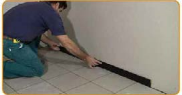
Apply ceramic or wood baseboard to the wall above the Profyle Flat
