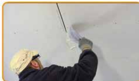
Fill the possible gaps between panels
