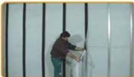
OPZION - STYWALL STRIPS: Apply the adhesive Stywall strips on the boards side of vertical metal studs
