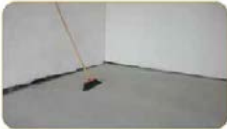
Clean the applying surfaces from dirty and sharp parts
