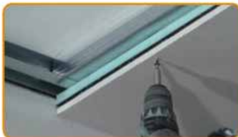
Fix the Rewall panel to the metal frame with 55 mm screws every 15 cm
