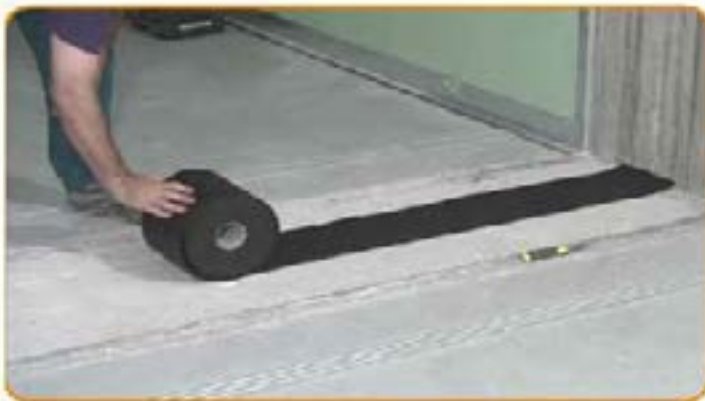
Lay the under wall strip
