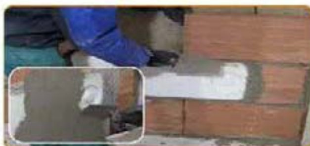
Build the wall around the Sylencer and plaster using a specific mesh.
