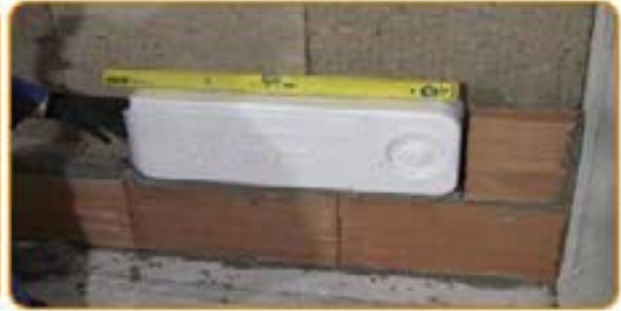
Lay on mortar the Sylencer
