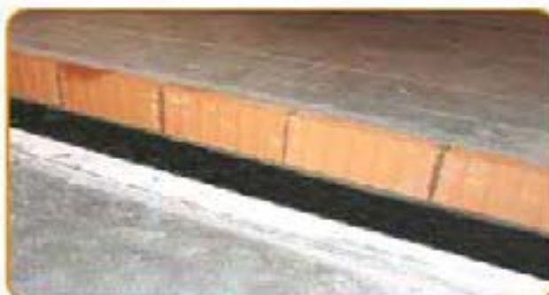
Realize brick wall on the strip, applying it on the mortar layer.
