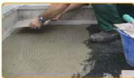
Spread the bi-component concrete glue, layer the ceramic tiles over the adhesive glue.
