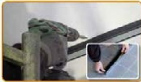
Glue the adhesive strip Stywall S3A to the metal studs and fix them along the perimeter of the room at a fixed distance from the
