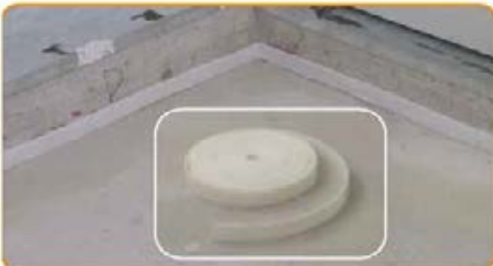
Fix the Profyle Flat 5 around the bottom of the surrounding walls
