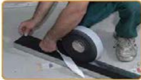
Glue on the metal studs the adhesive strip type Stywall S3-A
