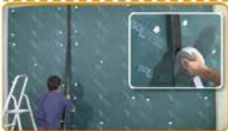
When all panels are fixed seal the panel joints with the "Stik" tape.
