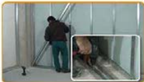
OPZION - DOUBLE STRUCTURE - Built up the second metal studs structure.
