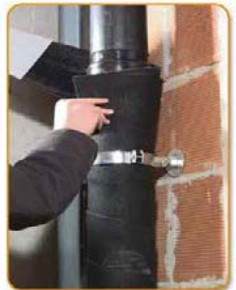
Carry on the installation of the pipes.
