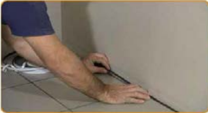
Remove the protective film and glue the strip along the perimeter of the room
