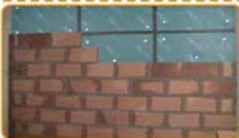
Build up the second wall by caring to joint the blocks with mortar on both vertical and horizontal joints.
