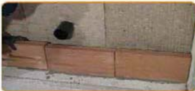
Start the building of the wall and stop at the height decided for the ventilation hole.
