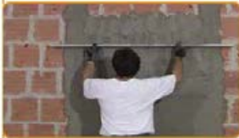
Apply in the first wall a layer of row mortar of about 1 cm thickness.
