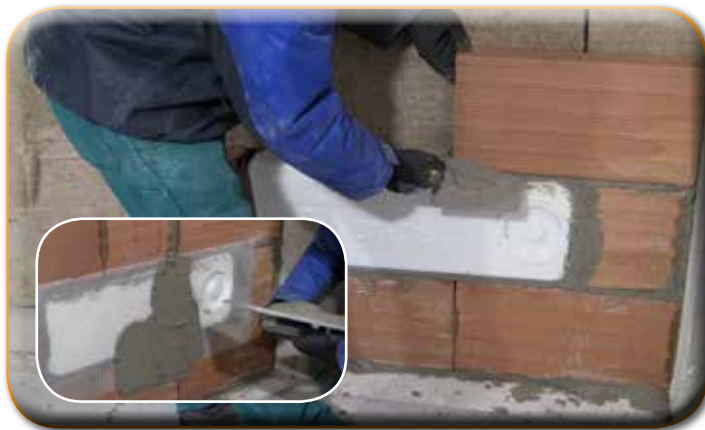
Realizzare la parete attorno al Sylencer e intonacare utilizzando la rete portaintonaco Build the wall around the Sylencer and plaster onto the product with a plastic mesh
