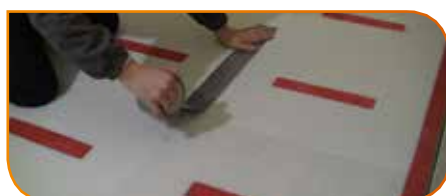
Sigillare eventuali fessure tra i componenti mediante il nastro Stik Seal any gap between two adjacent components with Stik tape
